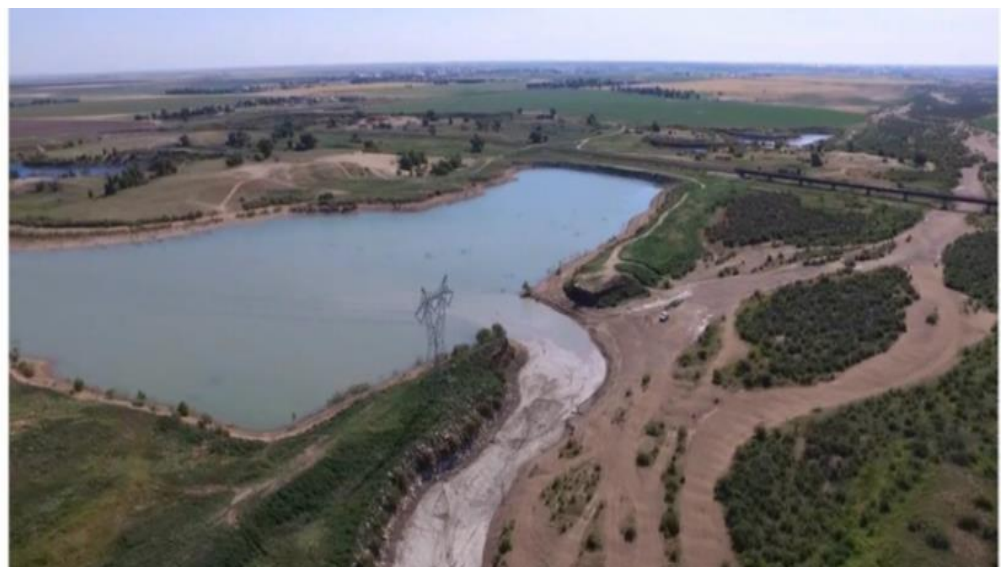
Figure 7. Ark River breach in state riverbank property upstream of Garden City.
